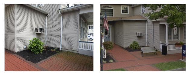
A downspout planter box can be installed near the west entrance of the building to capture the stormwater from the downspout. A rain garden can be installed in the turfgrass area by the walkway to the east of the building to capture, treat, and infiltrate the stormwater runoff from the nearby parking lot.
