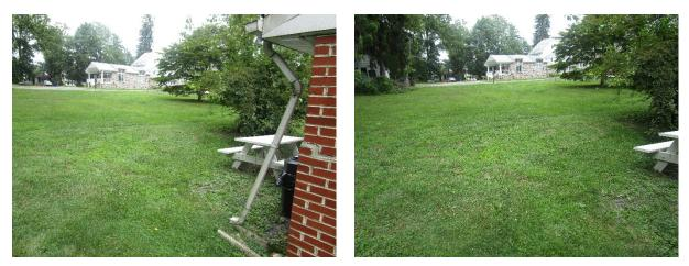
A rain garden can be installed in the turfgrass area located at the northwest corner of the library by allowing the disconnected downspout to flow into the garden to capture rooftop runoff. The runoff would be filtered naturally as it permeates the ground through the rain garden. A preliminary soil assessment suggests that more soil testing would be required before determining the soil's suitability for green infrastructure.
